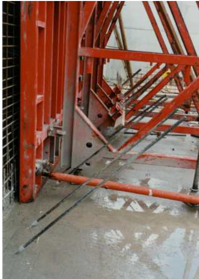
suspension frames, reanchored in correct angularity of 45°
