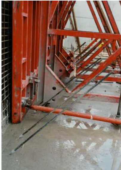
suspension frames, reanchored in correct angularity of 45°
