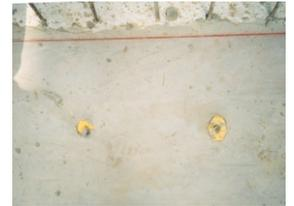
The "EhS Anchors" are supplied with a PE-45° Recess
