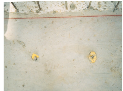
Anchor Position before removing Recesses
