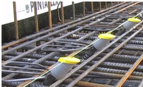
Recesses leveled by a string
