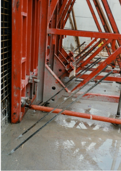
Suspension Frames, reanchored in correct angularity 45°
